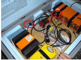
12. Connect timing antenna (TIMING-GPS ANT.) bulkhead cable to GPS ANT. port on seismic logger (Q330).
