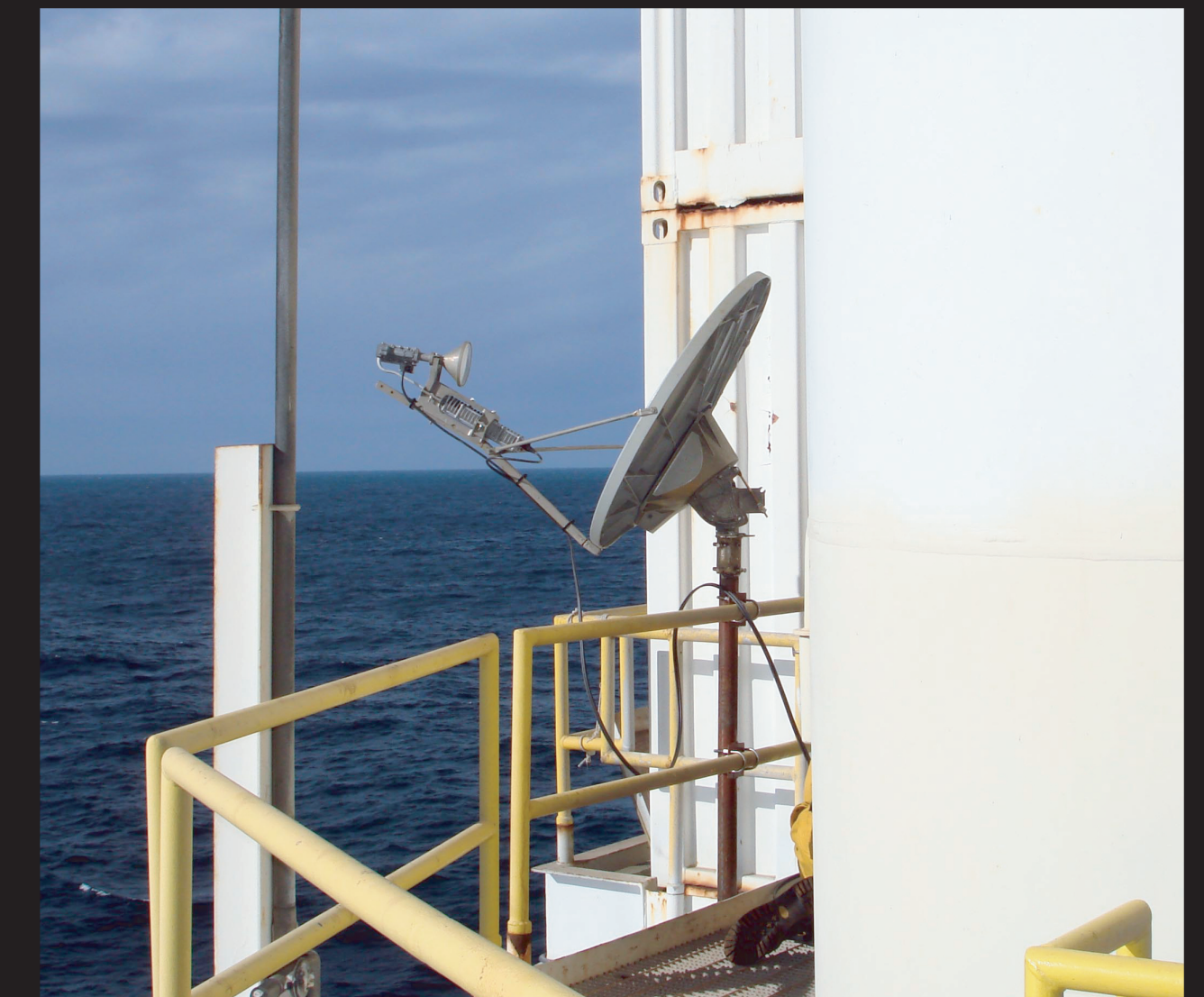
VSAT communications system on Harvest Oil Platform. VSAT provides internet for the various scientific instruments aboard the platform.
